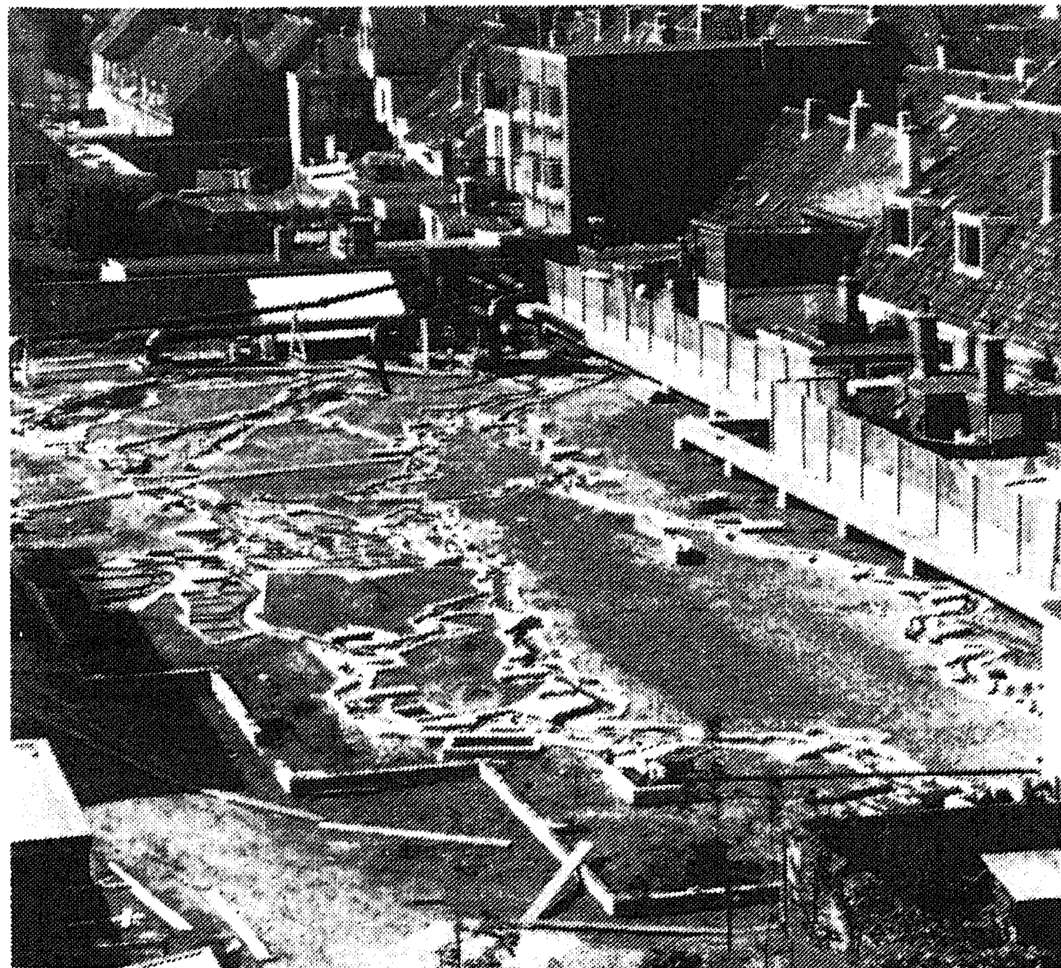
FIGURE 3. The construction of the scale model, about 1948 (Photo: Waterloopkundig Laboratorium Delft).
